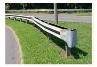
Figure 6-2: Blunt Guardrail Terminal
