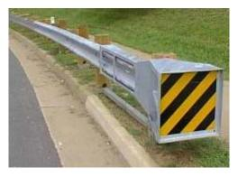
Figure 6-3: Sequential Kinking Terminal and Energy Absorption Barrier
